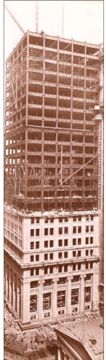
BANKERS TRUST BUILDING Construction Photograph, April 11, 1911
